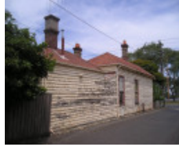
Edwardian Dwelling - West Facade
