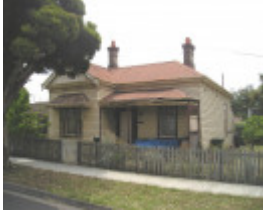
Edwardian Dwelling - Main Facade (South Elevation)
