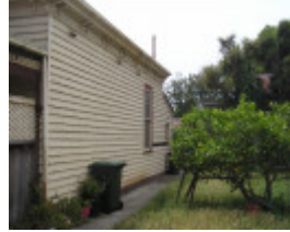
Edwardian Dwelling, East Facade
