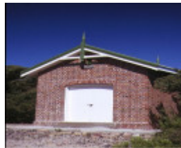
new works lakes entrance rocket shed
