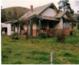
Orchard House 25 Cottles Bridge - Strathewen Road Cottles Bridge Colour 1 - Shire of Eltham heritage Study 1992
