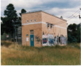
Wattle Glen railway 50hz electricity substation Colour 2
