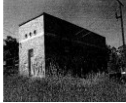
Wattle Glen railway 50hz electricity substation
