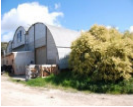
B5438 Former Quonset Hut
