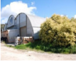
B5438 Former Quonset Hut
