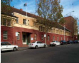
B6139 Former Royal Australian Army Medical Corps Training Depot
