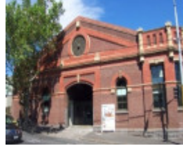
B3890 Fmr Cable Tram Engine House Nth Melbourne
