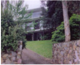
B6035 Delbridge House
