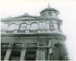
B3404 Former Kensington Property Exchange
