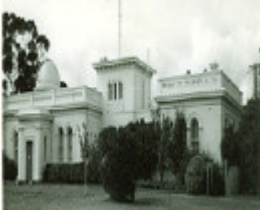
B0411 Observatory Building Melbourne
