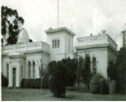
B0411 Observatory Building Melbourne
