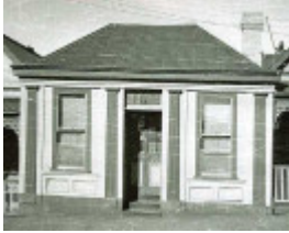
B0348 Builders Inn
