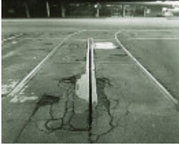
B5088 Cable Tram Tracks
