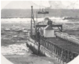
New Works, Lakes Entrance
