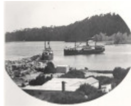
New Works, Lakes Entrance
