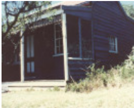
New Works cottage
