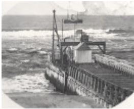
New Works, Lakes Entrance
