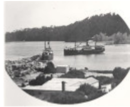
New Works, Lakes Entrance
