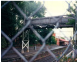
B6321 Middle Brighton Footbridge
