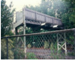
B6321 Middle Brighton Footbridge
