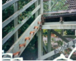
B6321 Middle Brighton Footbridge
