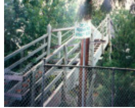
B6321 Middle Brighton Footbridge
