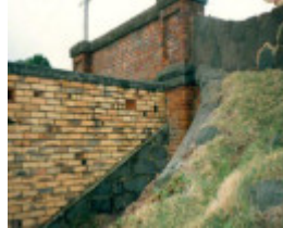
B2065 Tunnel Station to Pier
