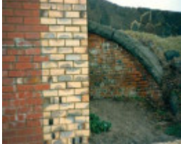
B2065 Tunnel Station to Pier
