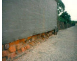
B2065 Tunnel Station to Pier
