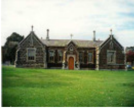
B1028 St Andrews School House
