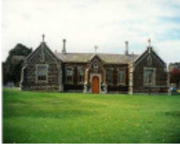
B1028 St Andrews School House
