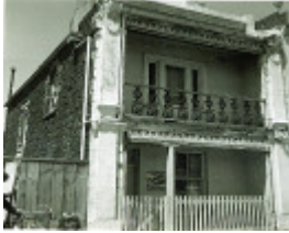
B3822 Terrace House
