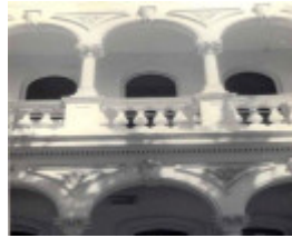
B3648 Exterior Detail
