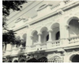
B3648 Upper Balconies
