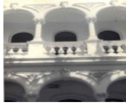
B3648 Exterior Detail
