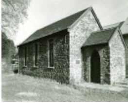
B4820 Former St John the Less Church
