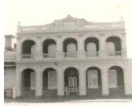
B0812 111 Chapman St North Melbourne
