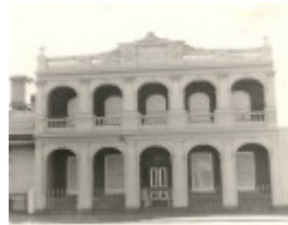
B0812 111 Chapman St North Melbourne
