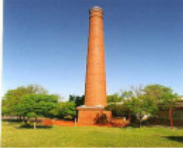
B6871 Boiler House Chimney
