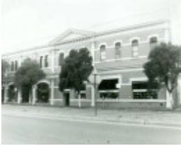
B6141 115 143 City Road Southbank
