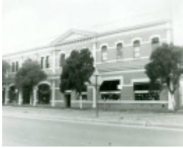
B6141 115 143 City Road Southbank
