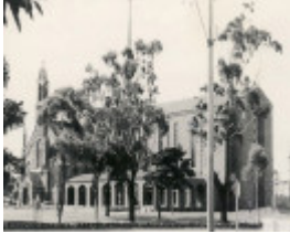
B1027 St Andrews Anglican Church New St Brighton
