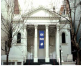
B0082 Collins Street Baptist Church
