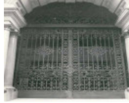
B3331 Fmr Commercial Bank of Australia Gateway
