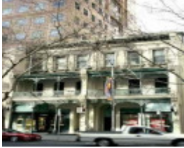
B3920 Terrace Houses
