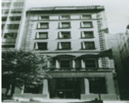
B4331 Former London & Lancashire Building
