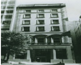
B4331 Former London & Lancashire Building
