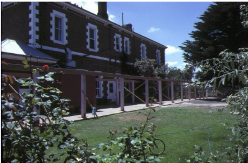
pirra homestead windermere road lara rear walkway & pergolas jan1985
