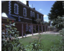
pirra homestead windermere road lara rear walkway & pergolas jan1985
