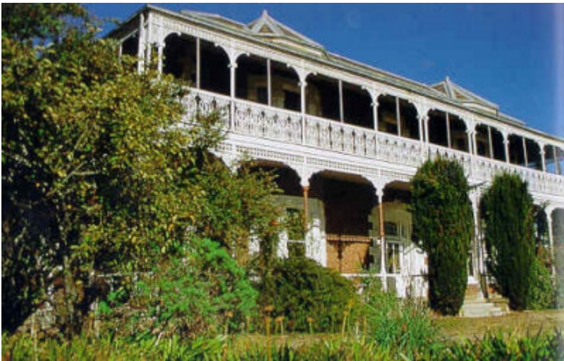
pirra homestead windermere road lara front view publication
