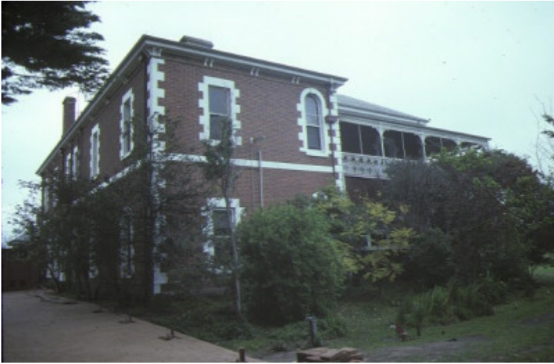
pirra homestead windermere road lara side view sep1984
