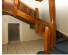
B4908 Canterbury Mansions Entrance Stairway
