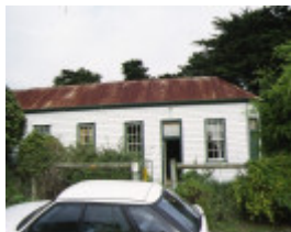
1 former wattle hill hotel lavers hill front view april 1994
