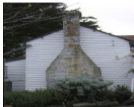
former wattle hill hotel lavers hill side view & chimney april 1994
