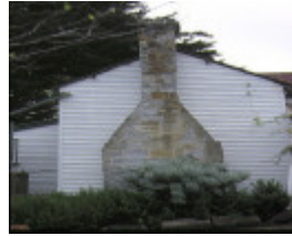
former wattle hill hotel lavers hill side view & chimney april 1994
