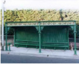
B7039 Cast-iron Tram Shelter
