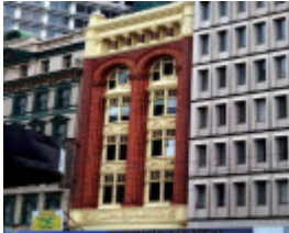
B4618 Paton Building
