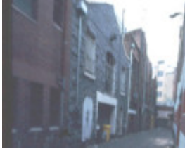
B6125 Heape Court Warehouses
