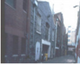
B6125 Heape Court Warehouses
