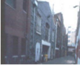
B6125 Heape Court Warehouses
