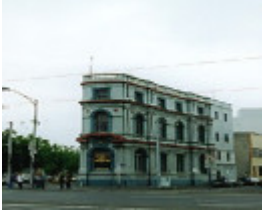
B6974 Former Colonial Bank
