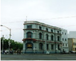
B6974 Former Colonial Bank
