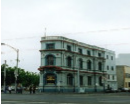
B6974 Former Colonial Bank
