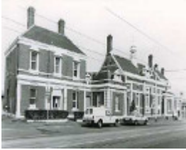
B5560 Court House & Police Station
