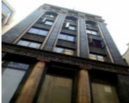
B4046 Majorca Building
