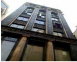
B4046 Majorca Building
