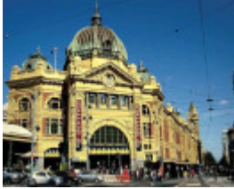
B3006 Flinders Street Station
