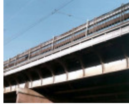
B5747 Flinders St Rail Viaduct
