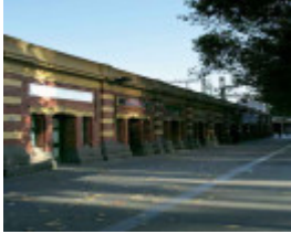
B5747 Railway Viaduct
