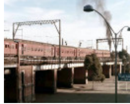
B5747 Flinders St Rail Viaduct
