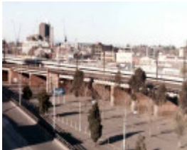
B5747 Flinders St Rail Viaduct
