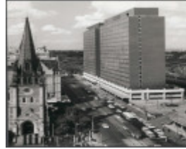
B6783 Gas & Fuel Buildings
