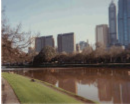
B6783 Gas & Fuel Buildings
