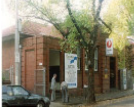
B6420 Former Post Office
