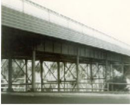
B1600 Metal Truss Bridge
