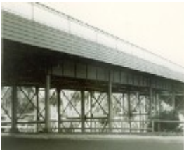
B1600 Metal Truss Bridge
