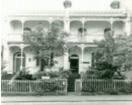
B4752 Terrace 62-64 Jolimont St East Melbourne.jpg
