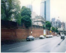
B6442 Retaining Wall
