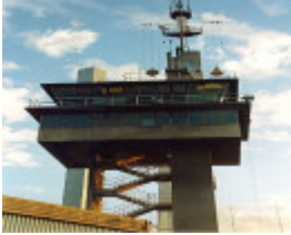
B7180 Shipping Control Tower
