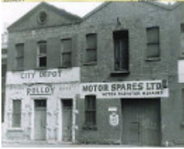
B1775 Commercial Warehouse North Melbourne
