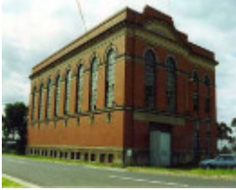
B3682 Albion Sub-Station
