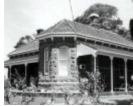
B1492 Green Hills NE Corner
