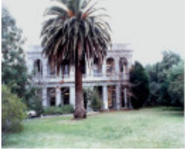
B0810 Former Blackhall
