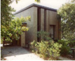
B6213 RG Lawrence House & Flats
