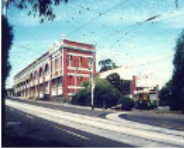
B6151 Tram Depot
